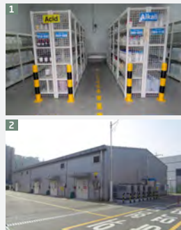
1 Separate storage and management of each chemical substance 2 Exclusive storage facility of chemical substances
